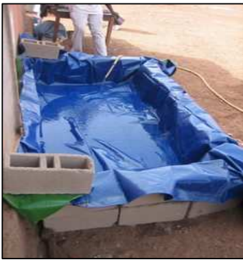
Water in the basin.
